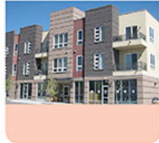
Mixed-uses with ground floor retail
