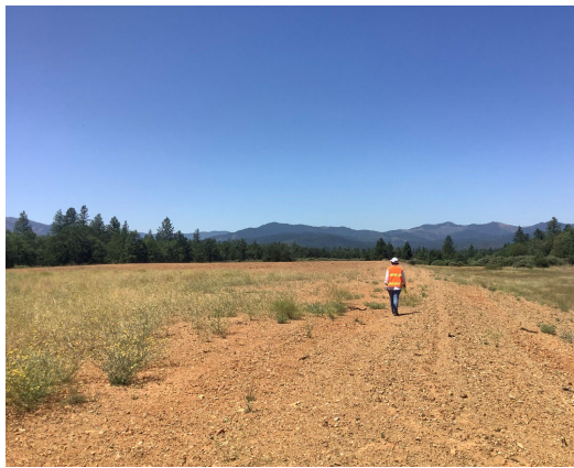
Photo 2. Looking north at the proposed runway extension area.
