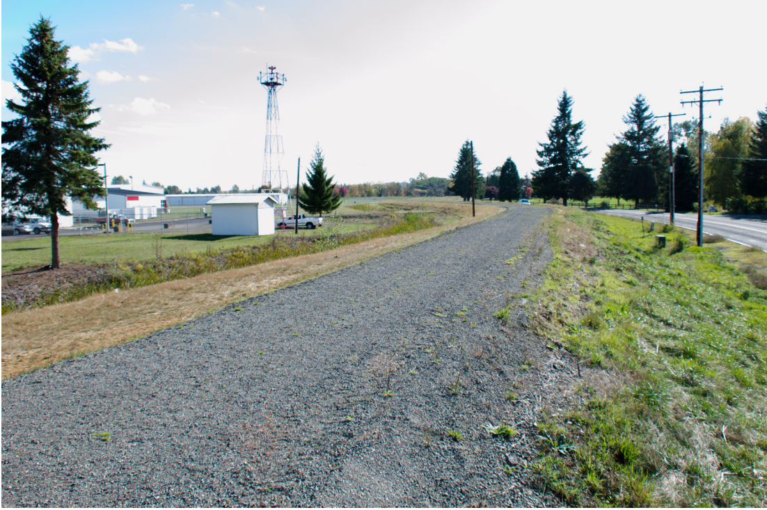
Typical View of the Airport Levee Improvements Project Area from the Existing Levee
