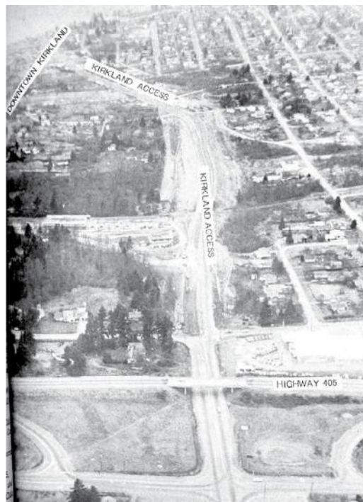
Construction of NE 85th Street
