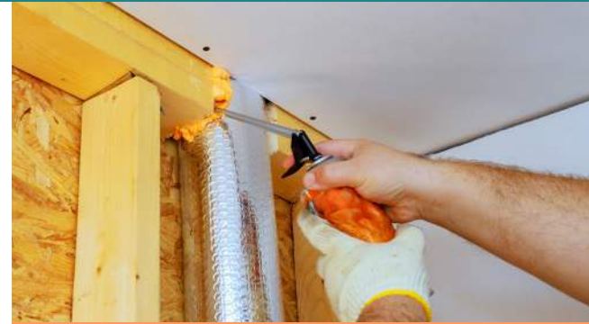
Air sealing improvements
